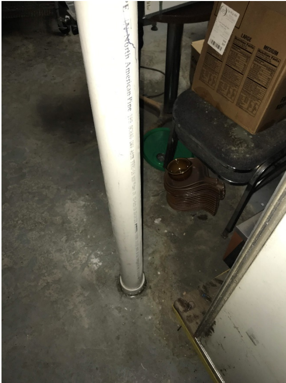
Photo 7: Floor at northern pickup point.
