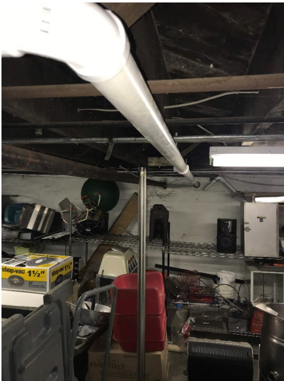
Looking south at lateral piping to southern pickup point.
