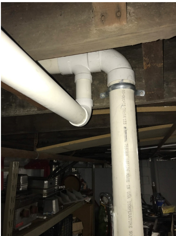
Photo 4: Looking east at northern pickup point and lateral to southern pickup point.
