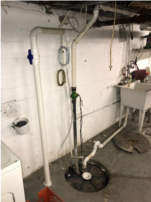
Photo 8: Looking northeast at southern pickup point (left side of photo) and sealed sump.
