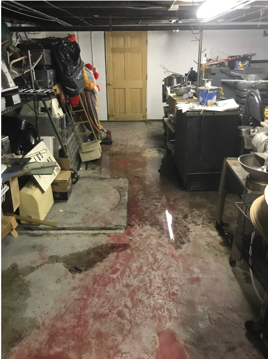
Photo 1: Looking west from near center south side of basement.
