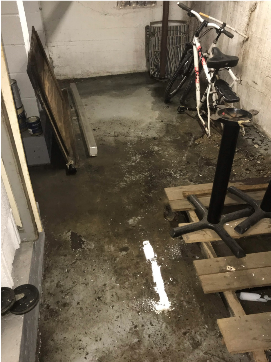
Photo 4: Looking at northeast corner of basement.
