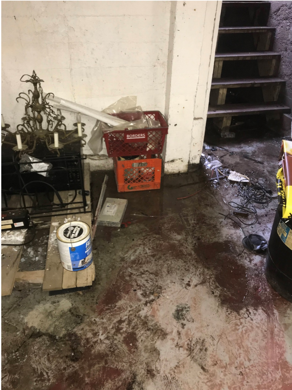
Photo 3: Looking east at east side entrance to basement.
