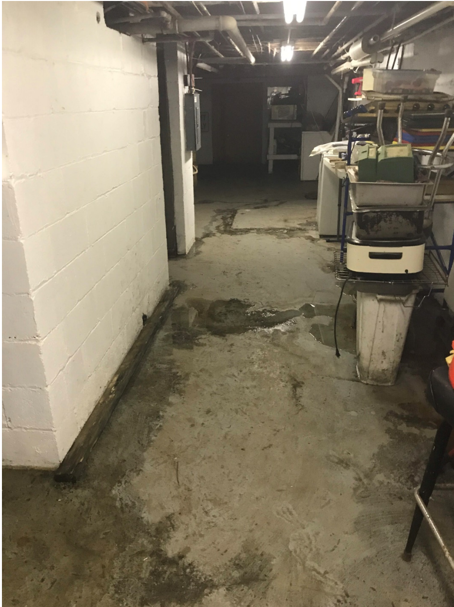
Photo 6: Looking west along south side of basement.
