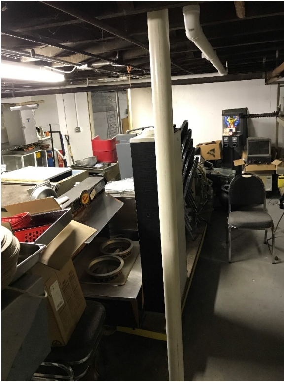
Photo 5: Looking west at northern pickup point and lateral piping to southern pickup point. 11/21/18
