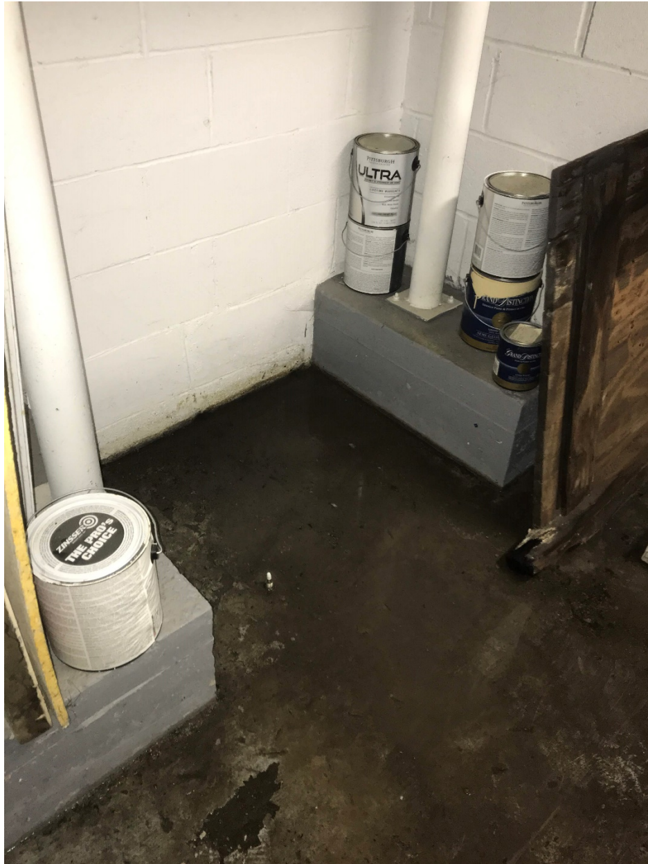
Photo 5: Looking at sub-slab port SS-3 at northeast corner of basement.
