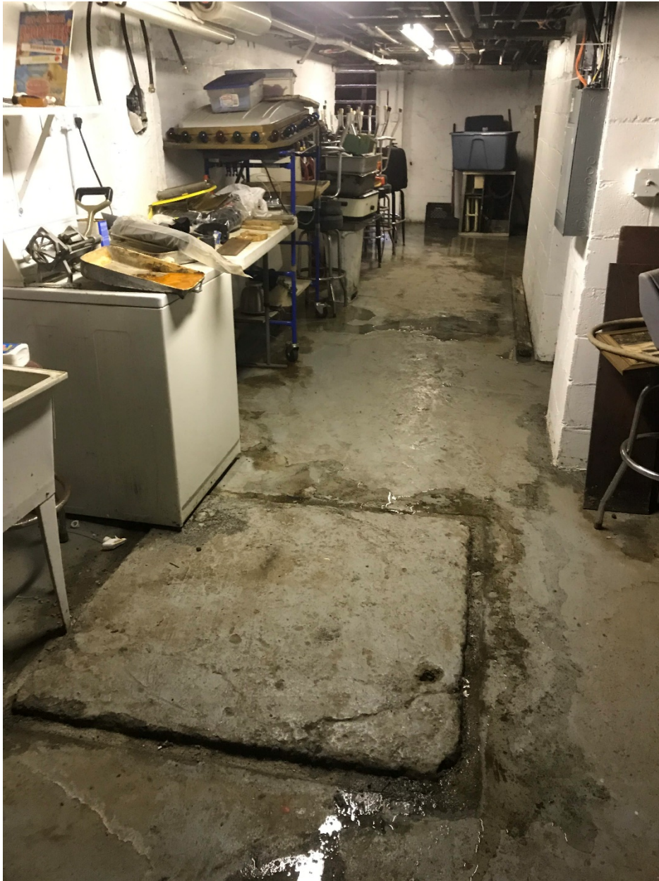
Photo 8: Looking east from south center of basement.
