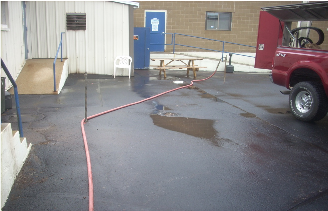
Photograph 4 Injection location near the building Date 15 June 2013
