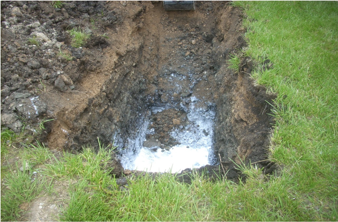
Photograph 1 Emulsified vegetable oil placed in excavated trench Date 10 June 2013
