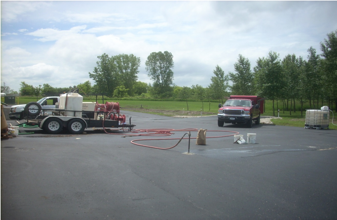
Photograph 3 Direct push rig and injection trailer showing connection to a well Date 24 June 2013
