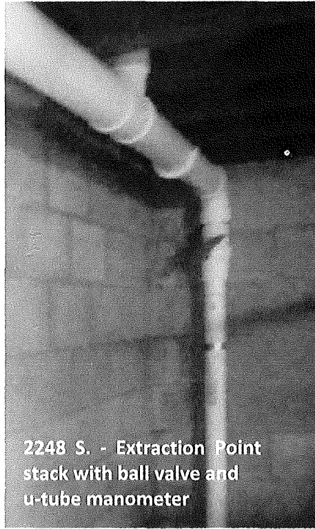
2248 S. - Extraction Point stack with ball valve and u-tube manometer.
