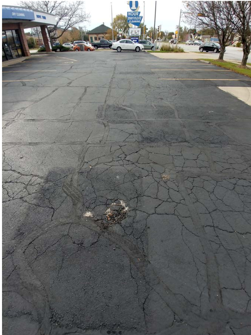
Asphalt condition in northern part of site – facing south
