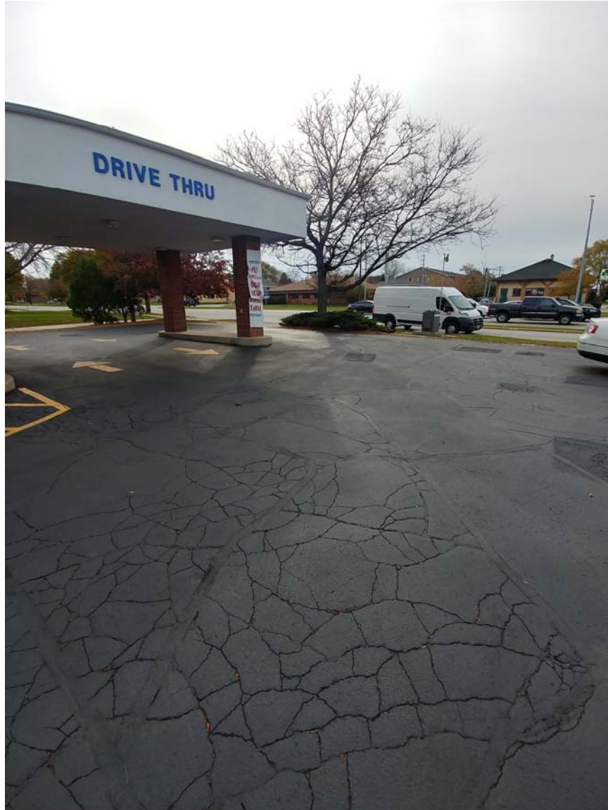
Asphalt condition in southern part of site – facing southeast
