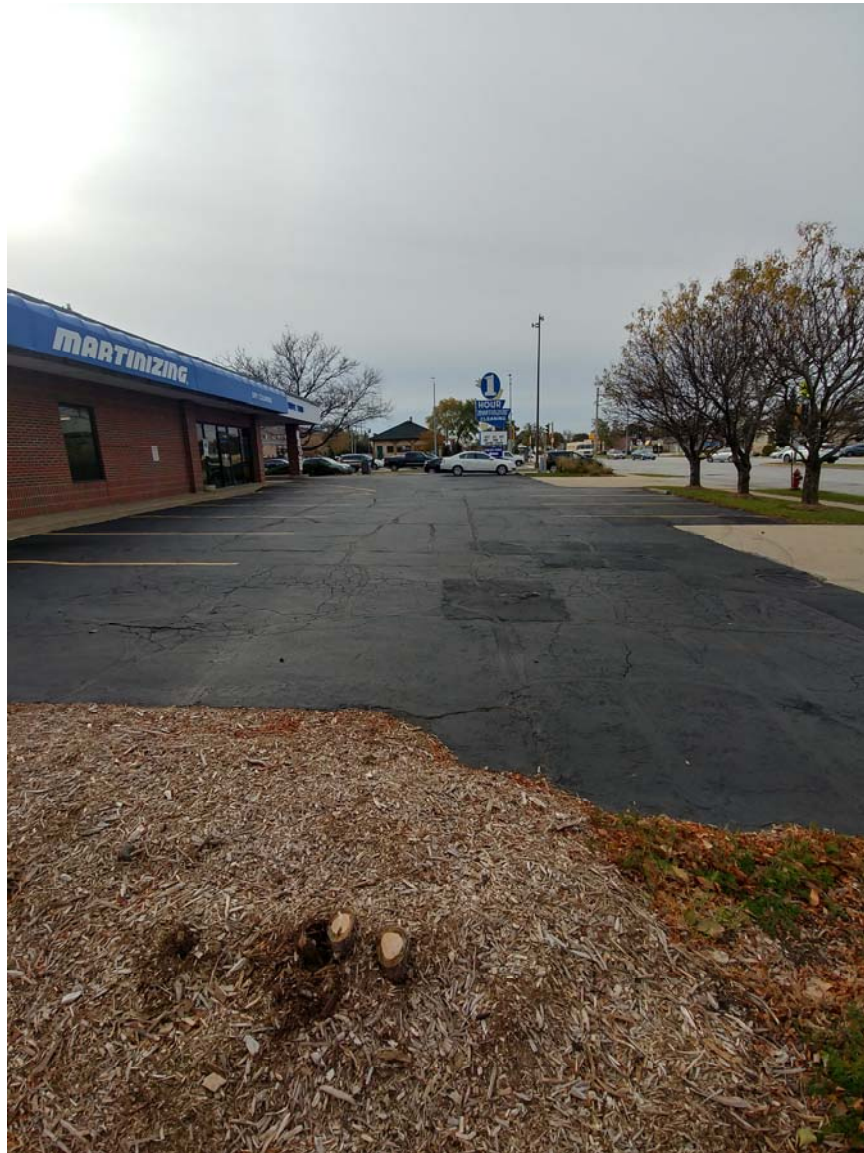
Overview of asphalt/concrete cap – facing south
