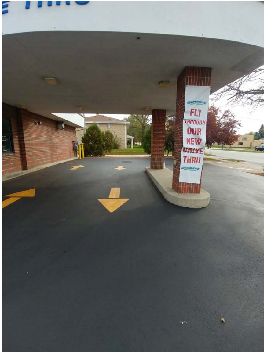
Overview of cap in drive-through area – facing east
