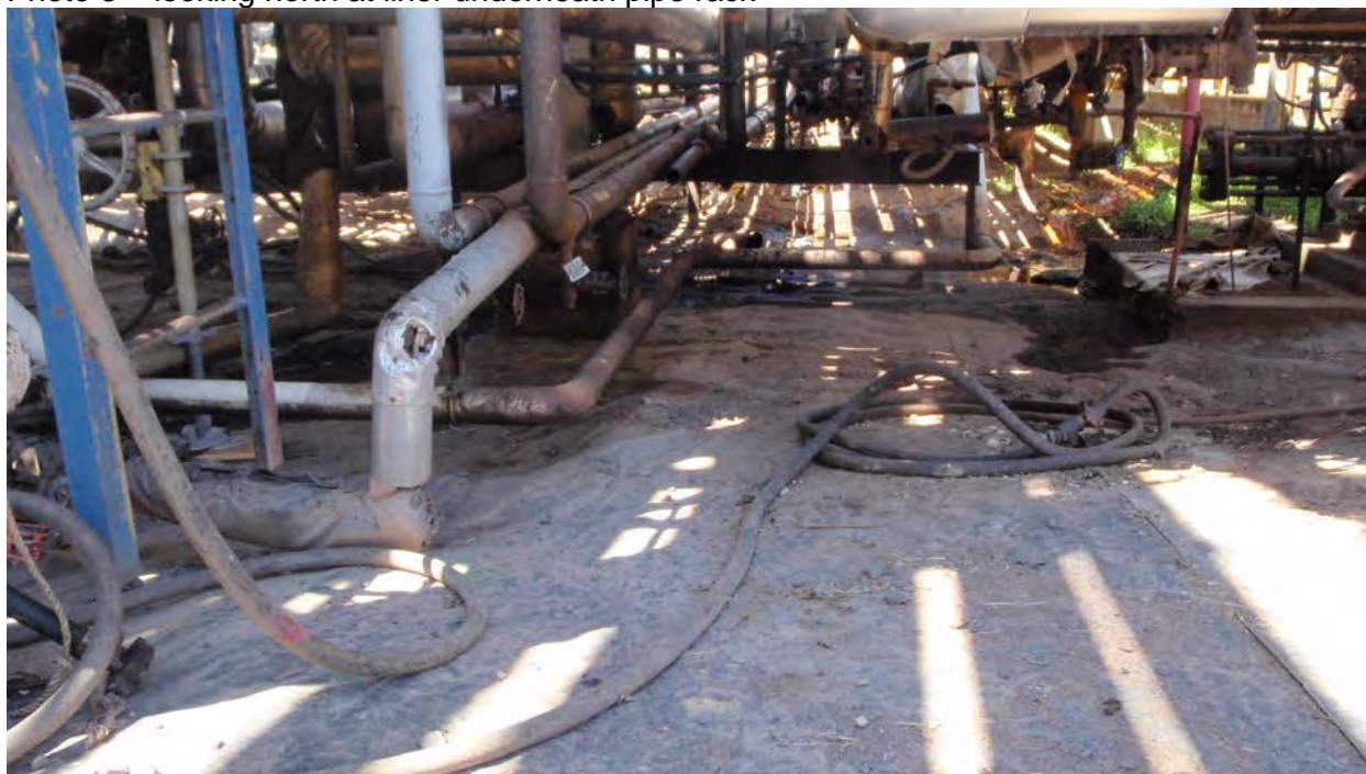
Photo 3 – looking north at liner underneath pipe rack
