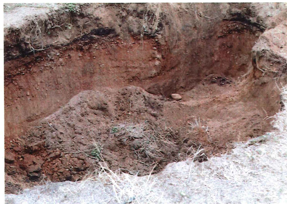
Photo 4 Tank Excavation Northwest Sidewall
