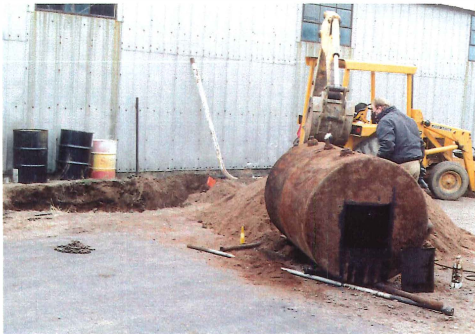
Photo 1 Removed 560 Gallon Diesel Tank
