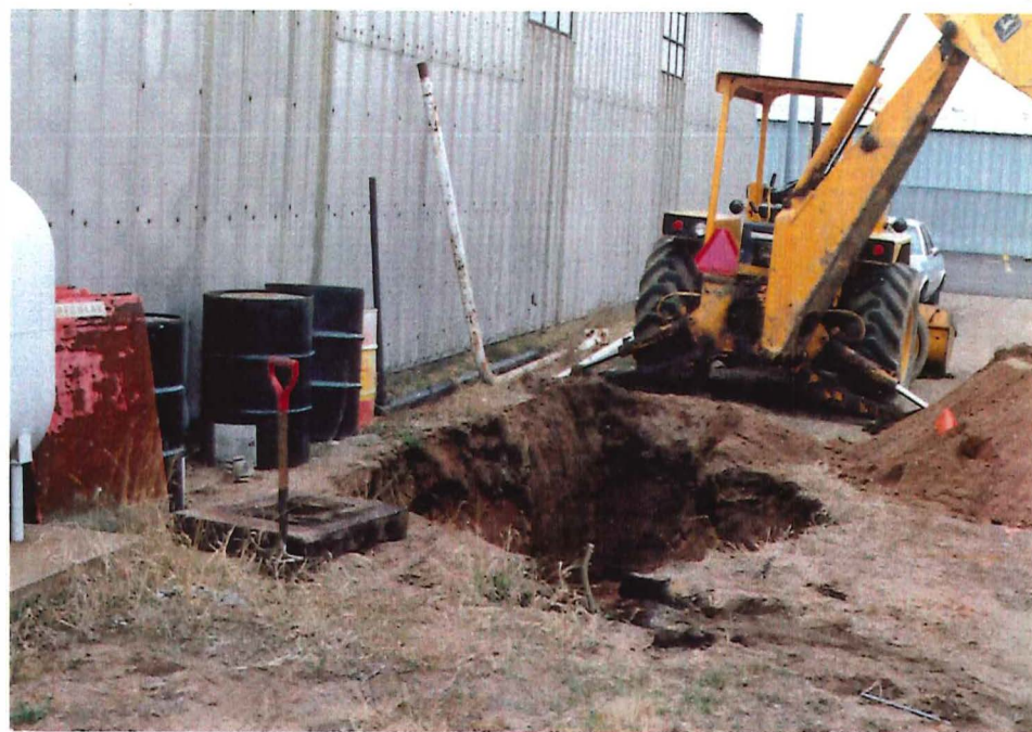
Photo 2 Tank Excavation
