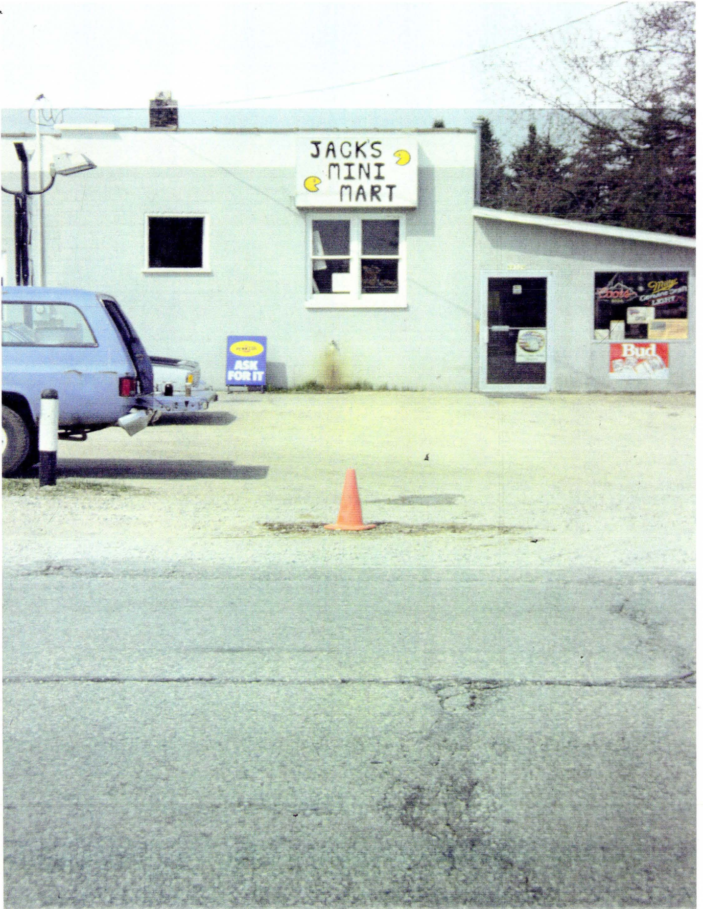
PHOTO 2 - LOCATION OF BORING B-1
