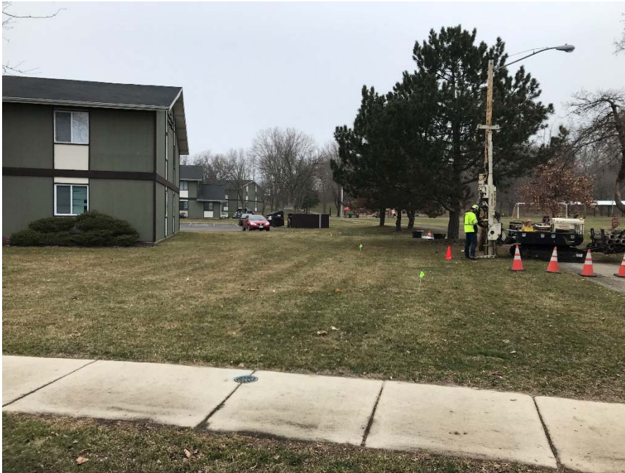
Photo 1: Looking north at installation of temporary soil gas sampling probe V-4 with V-3 in background. Green flags mark sanitary sewer.
