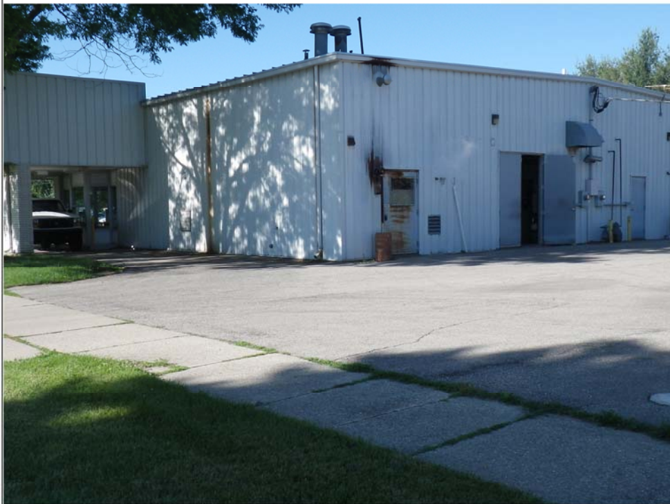
Title: Looking south southwest from east side of site.
