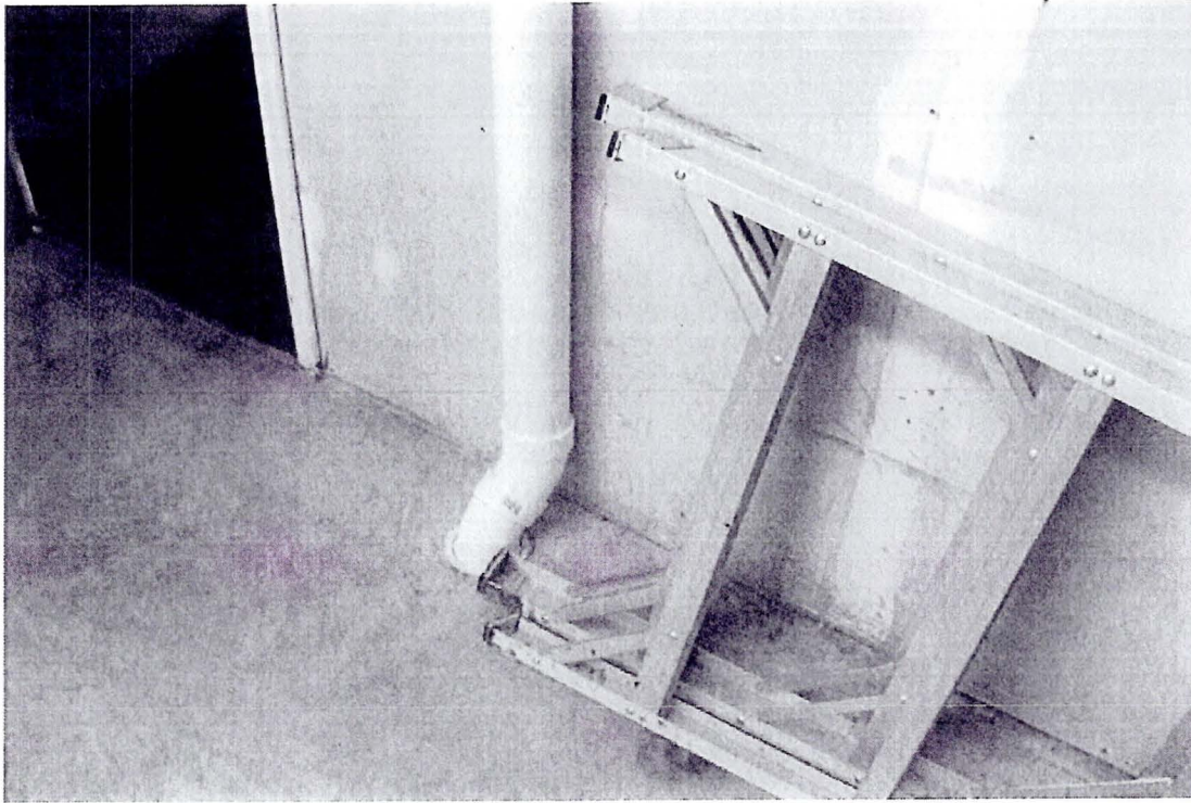
Photo 1 – front extraction point below concrete slab
