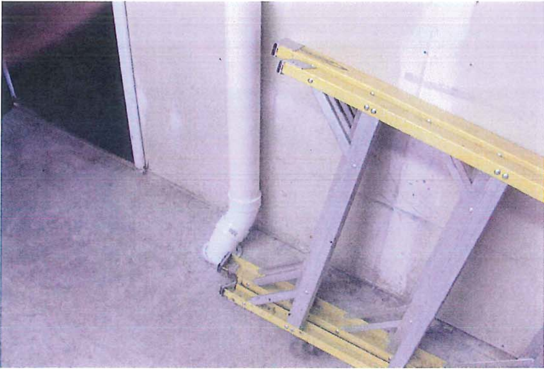
Photo 1 – front extraction point below concrete slab
