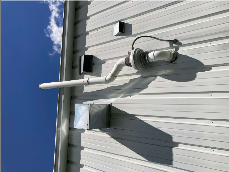
Title: Blower located on the west exterior of the building was operating.
