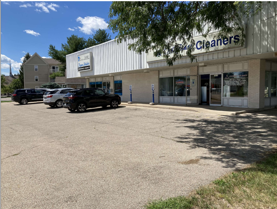
Title: Looking Northwest towards the building.
