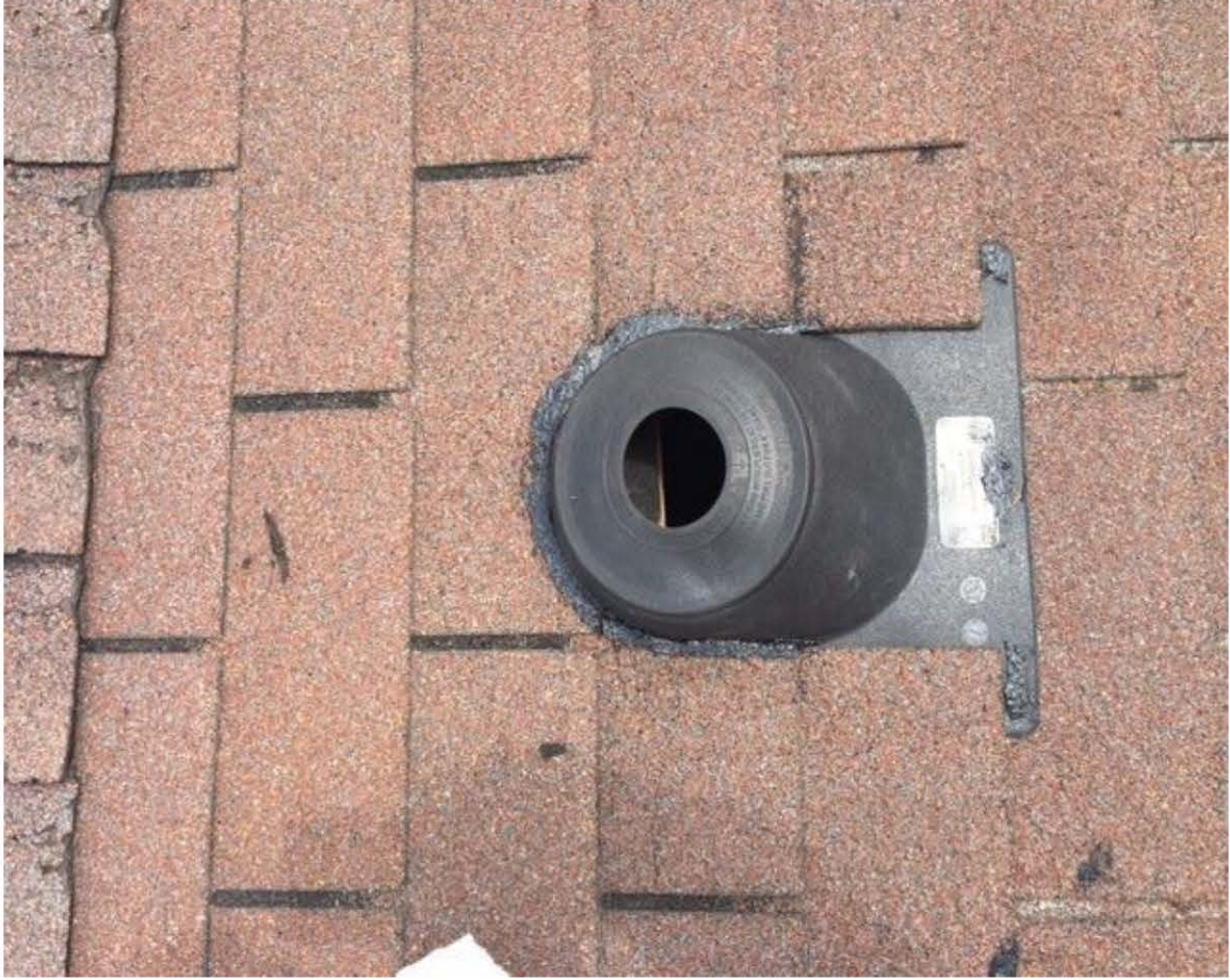
Penetration Point Through Roof of Attic - Exhaust Stack Not Yet Installed
