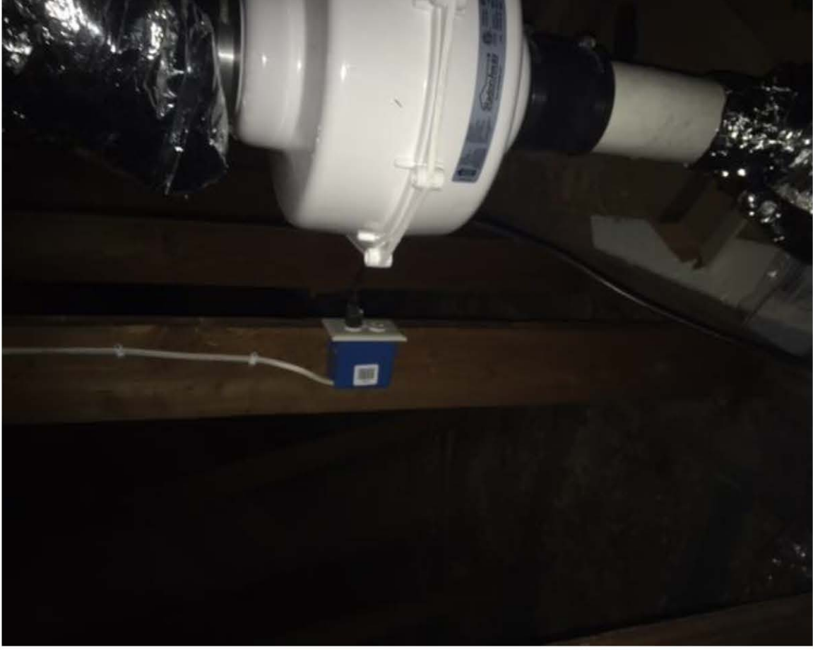
Dedicated Power for Depressurization Fan in Attic
