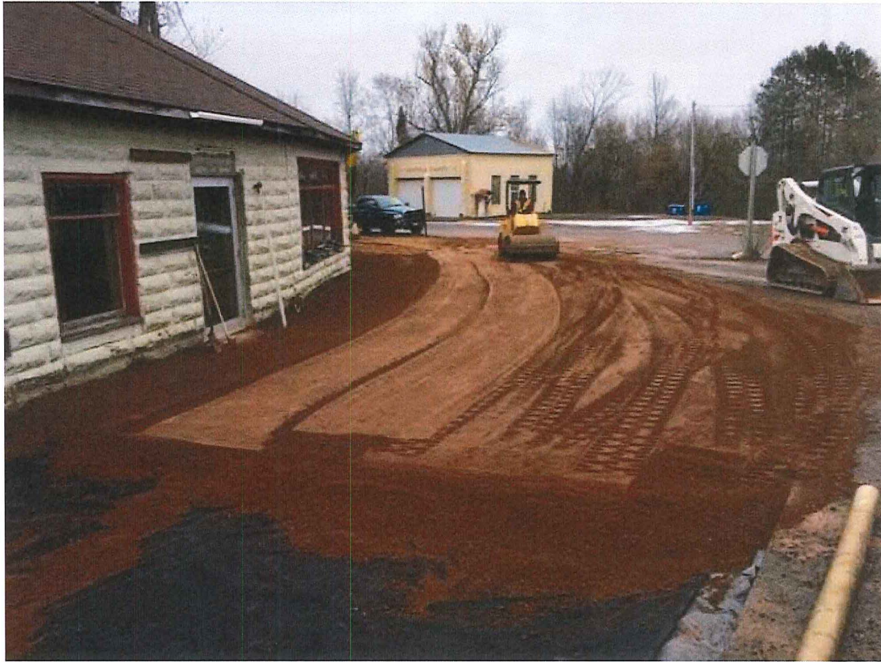
Sand over membrane
