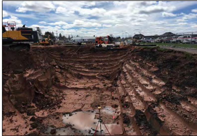
Completed UST excavation
