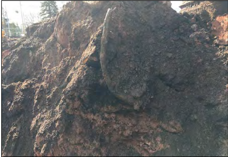
Buried pipe approximately 4' below land surface
