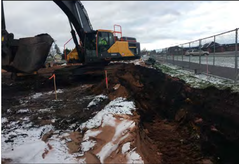
Excavating on north property line near B1
