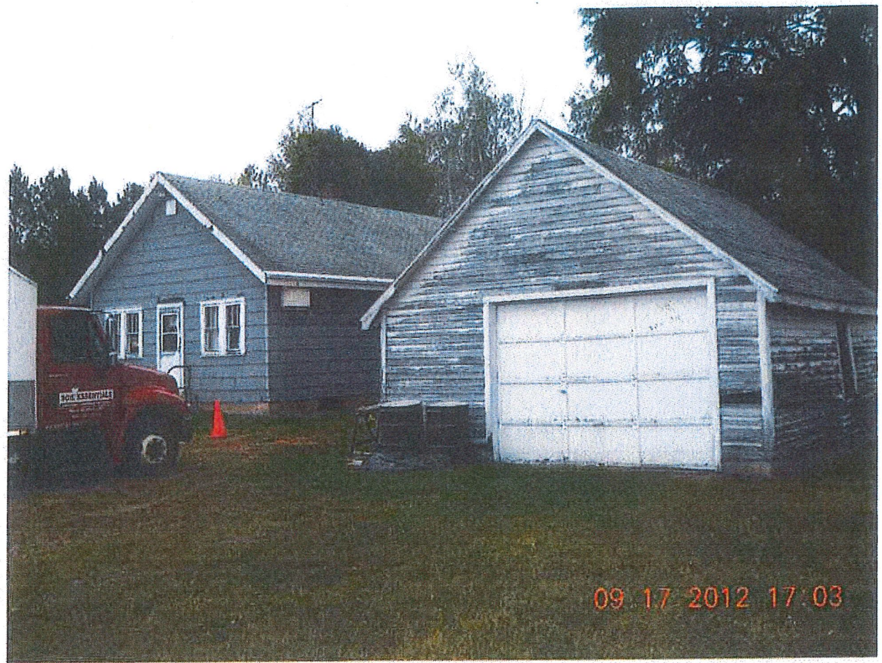
Photo #2: On site buildings (bar and garage) looking southeast
