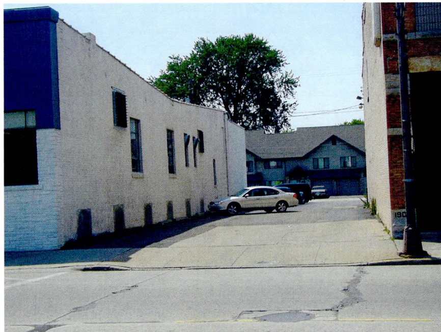
North side of building looking west from Main Street
