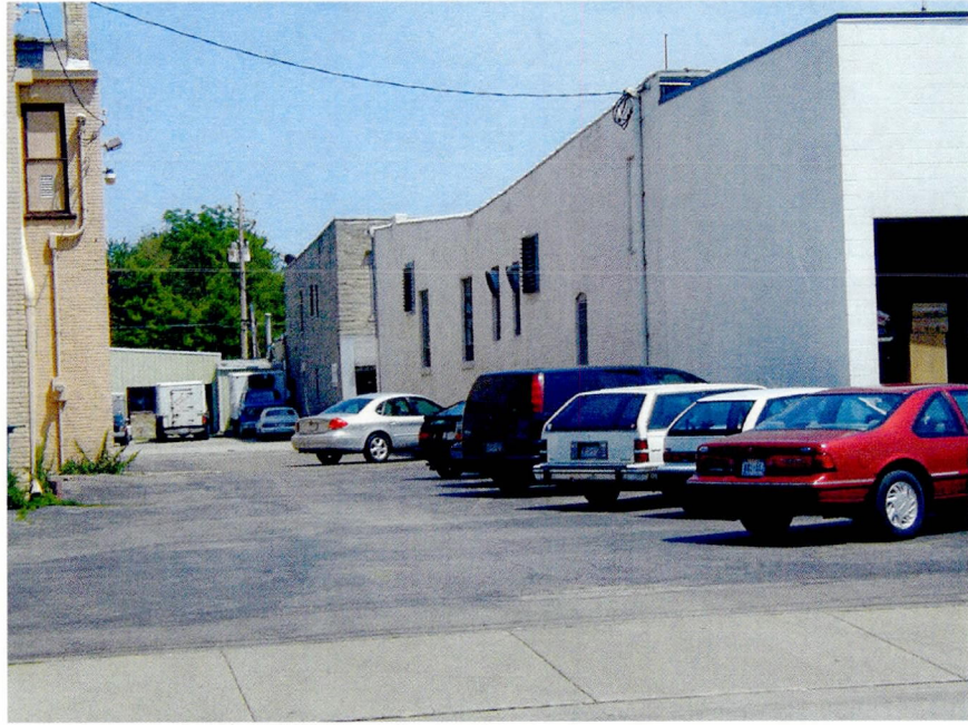
North side of building looking East from Division Street
