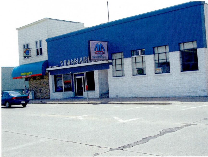
East side of Building looking west from Main Street – Front Entrance
