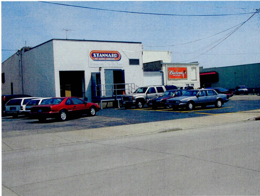
West side of building looking East from Division Street – Part of the existing cap
