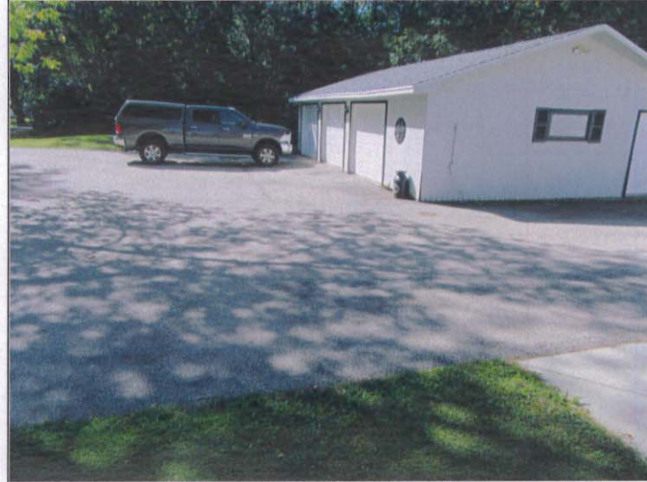
Title: View of cap area looking north to south (taken 9/12/2017)
