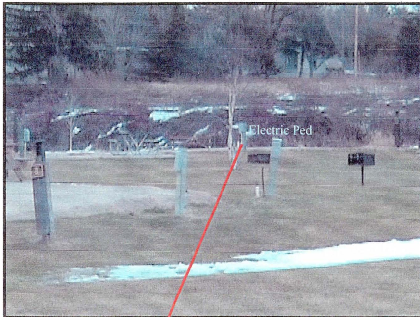
Figure 5 Line 00 for second survey January 10. Line runs from electric pedestal near lakeside through pedestal 225 out. Photo location noted on Figure 1.
