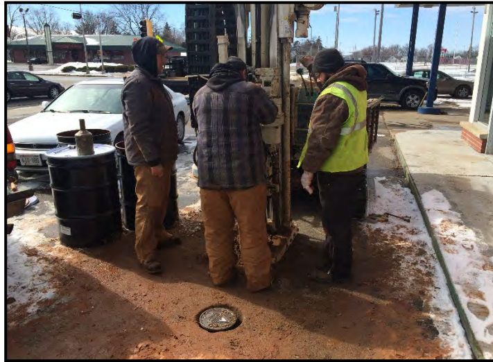
MW2r and CP4r Location
