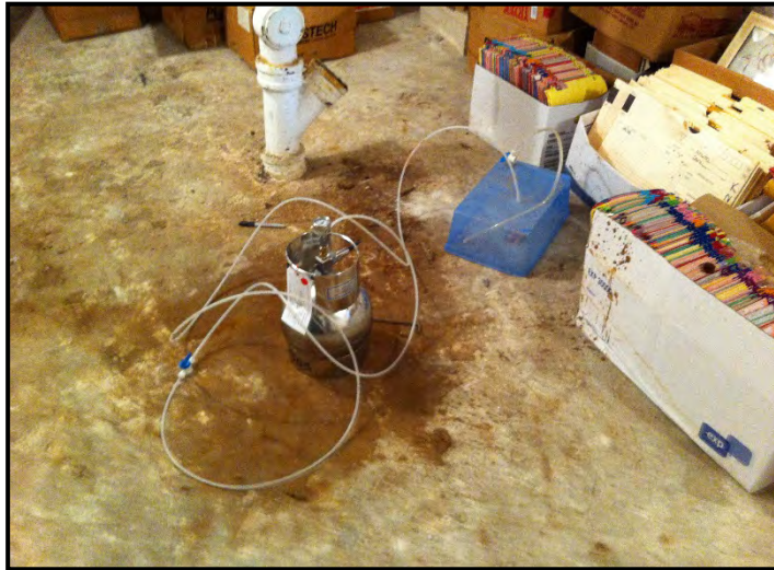
Sub-slab vapor sampling - Normington buiding, basement
