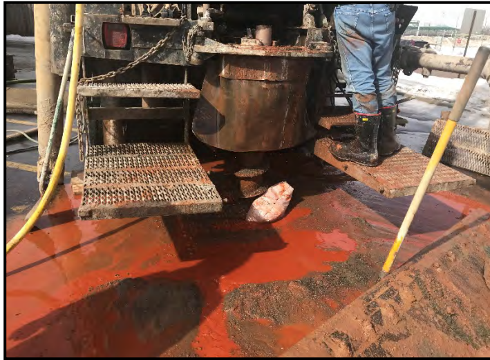
CPZ5D Air rotary drilling
