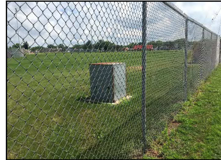
Witter Field sprinkler wells
