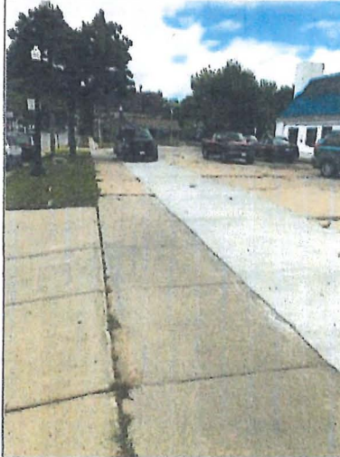
Title: Looking northeast at the area of concrete cap.
