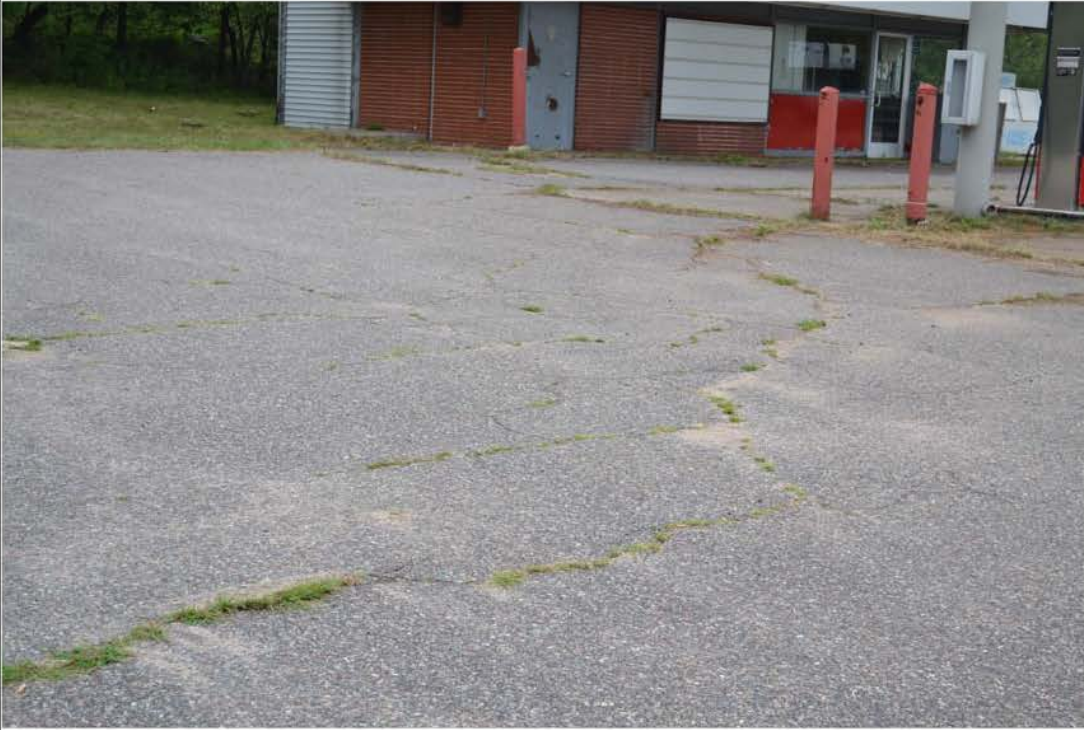
Title: Cap area close up. Photo is facing to the northwest
