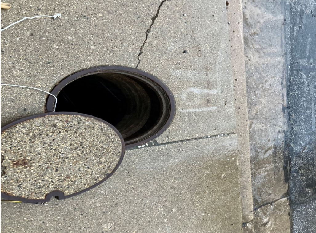
Photo 1: View of Sanitary Sewer Manhole 19 (IA-3) located along N. 32 nd Street.
