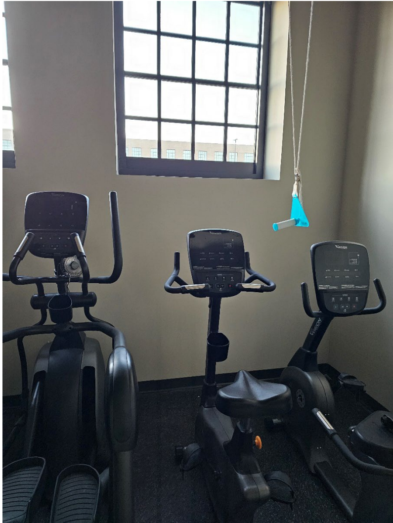
Photograph C-21. Room 1054 Fitness North Passive Sampler, EB-01-AV
