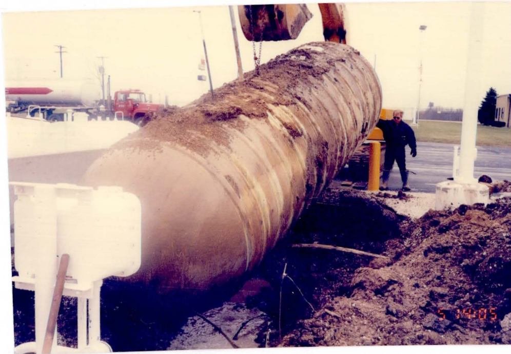
3. Removal of Additive UST.
