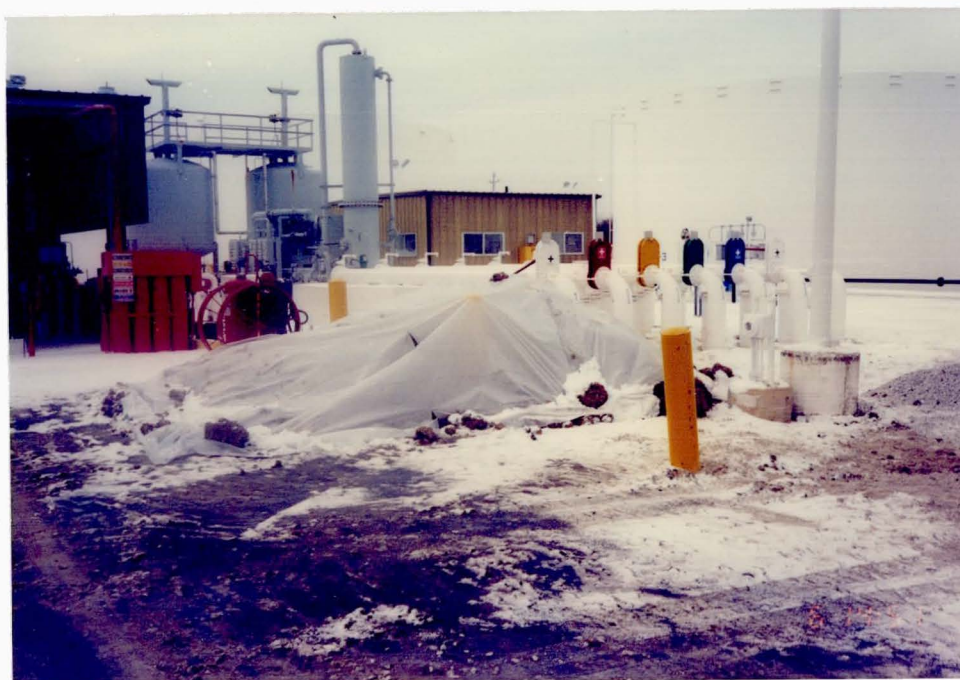
6. Stockpiled soils excavated from the surface in the UST area.
