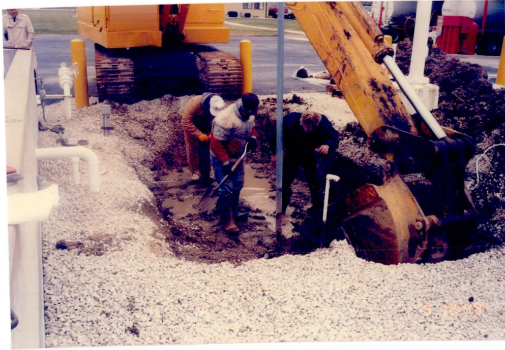
1. Schmidt Bros. personnel excavating soil from the top of the UST.
