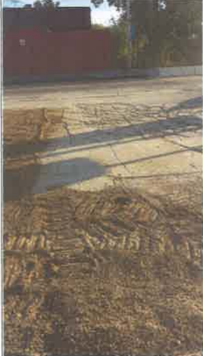
Title: Area of concrete cap to be maintained looking south.
