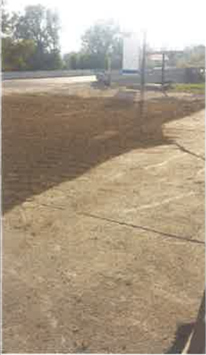
Title: Area of concrete cap to be maintained looking southwest.
