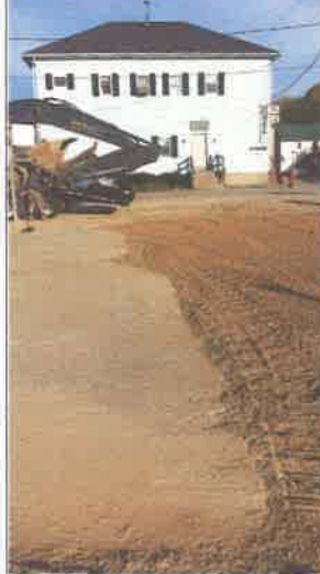
Title: Area of concrete cap to be maintained looking east.
