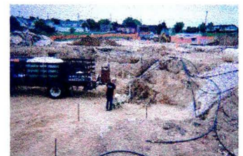
Photo Below: Initial carbon injection within partially backfilled excavation
