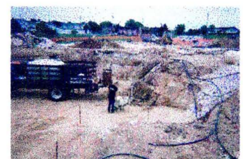
Photo Below: Initial carbon injection within partially backfilled excavation
