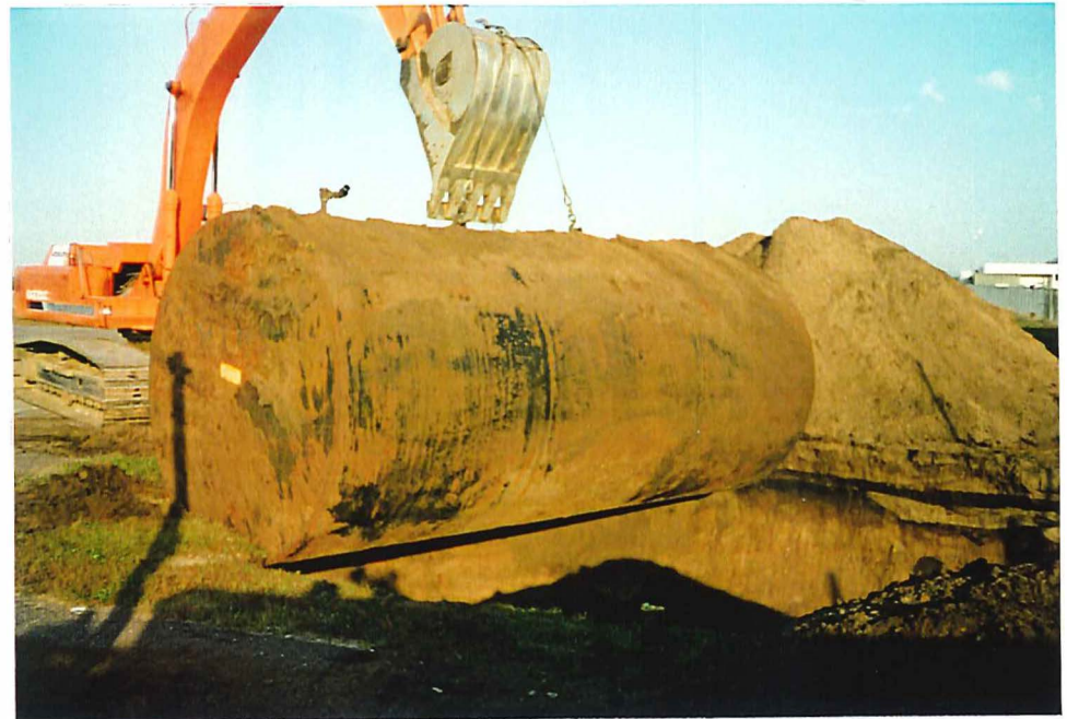
Photo 3 Heating oil UST being removed from ground
