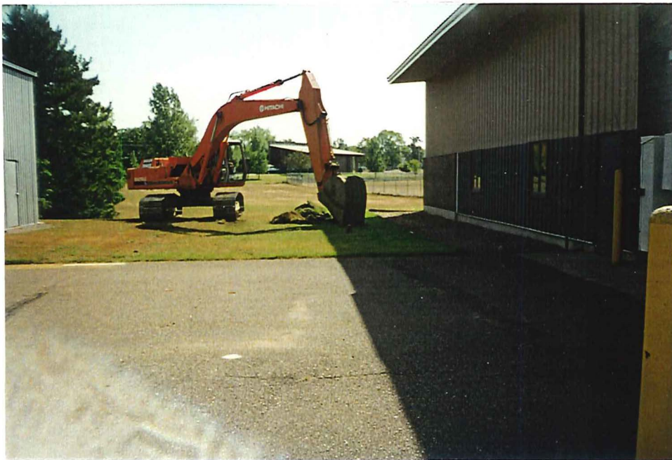
Photo 2 Heating oil UST area prior to excavation
