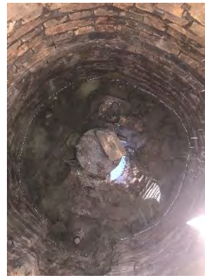
Site Photo- Inside of unknown manhole.
