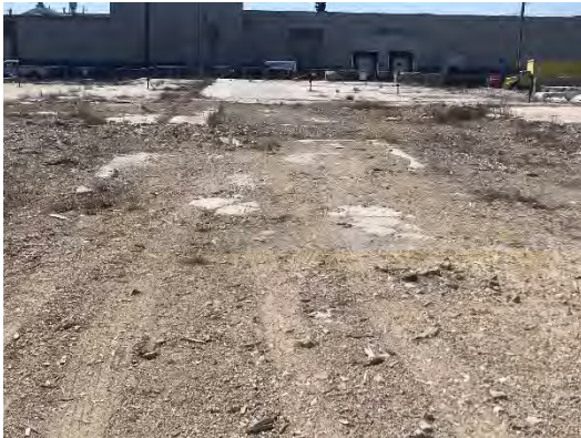
Site Photo- Tank Extents represented by yellow paint.
