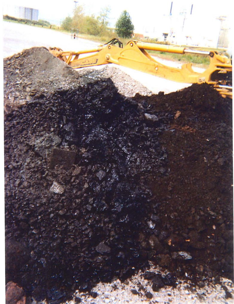
Photo 4: View of excavated material including soil, bricks, and cinders.
