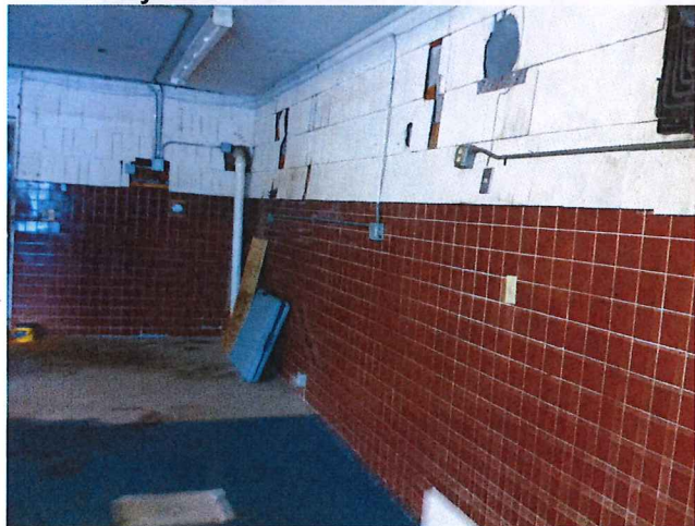
Internal System from S to N
