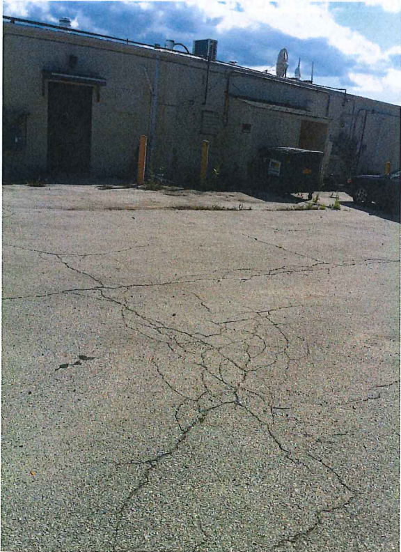
Asphalt Condition on N Side of Building
