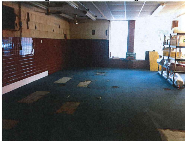
3 Monitoring Well Covers in Building from N to S
