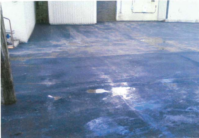
1. Asphalt engineered barrier behind K&W building looking north.
