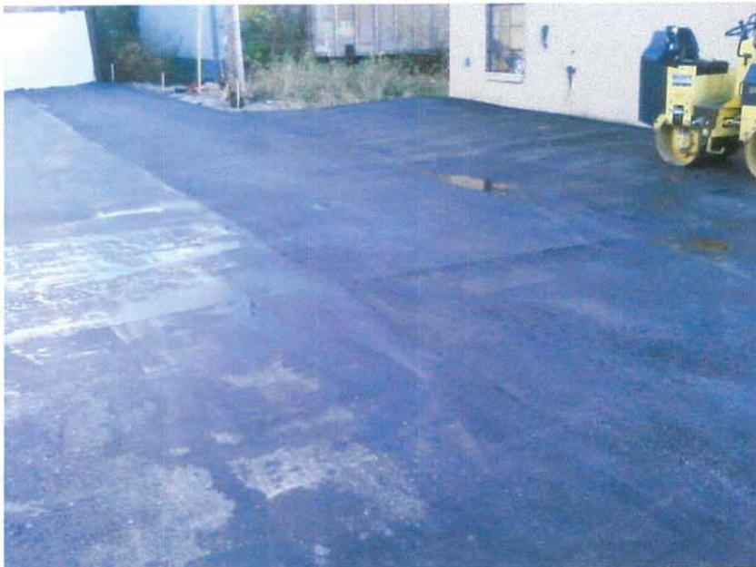
3. Asphalt engineered barrier behind K&W building looking south.
