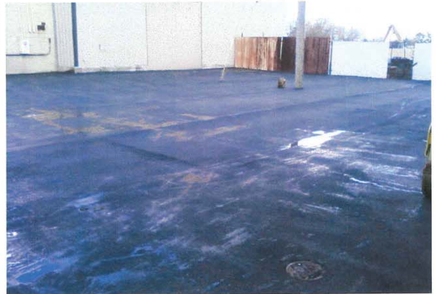
2. Asphalt engineered barrier behind K&W building looking west.
