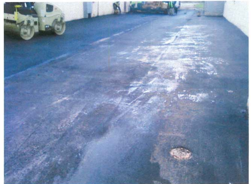
4. Asphalt engineered barrier behind former Key Products building looking east.
