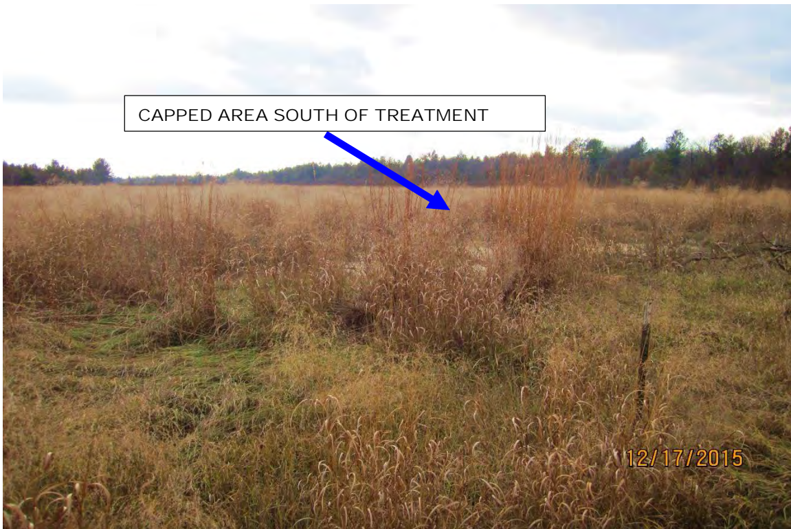
THE CAP CONSISTS OF A MINIMUM OF 18 INCHES OF CLEAN SAND, WITH MOST AREAS HAVING 22 TO 32 INCHES OF SAND. THE CAP IS VEGETATED WITH NATIVE PRAIRE GRASS. (VIEW IS TO THE SOUTHWEST)
