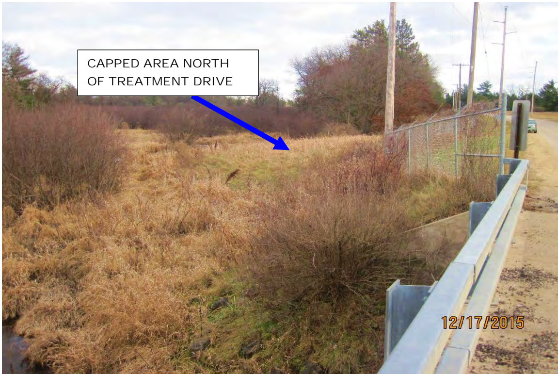
THE CAP NORTH OF TREATMENT DRIVE IS COMPOSED OF TWO FEET OF SOIL COVERED BY TOPSOIL WITH GRASS VEGETATION TO MINIMIZE THE POTENTIAL FOR EROSION (VIEW IS TO THE EAST)
