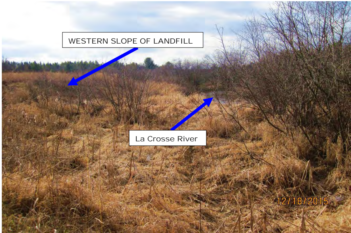
THE CAP OVER THE WESTERN SLOPE ALONG THE RIVER IS CONSTRUCTED OF 12 INCHES OF FILL OVERLAIN BY A GEOTEXTILE FABRIC, WHICH IS OVERLAIN BY 18-24 INCH RIPRAP ARMORING COVERED BY 2-4 INCHES OF SAND VEGETATED WITH NATIVE PRAIRE GRASS. (VIEW IS TO THE SOUTH)
