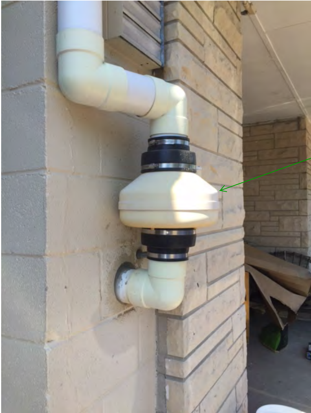
Vapor system located on the east side of the building.
