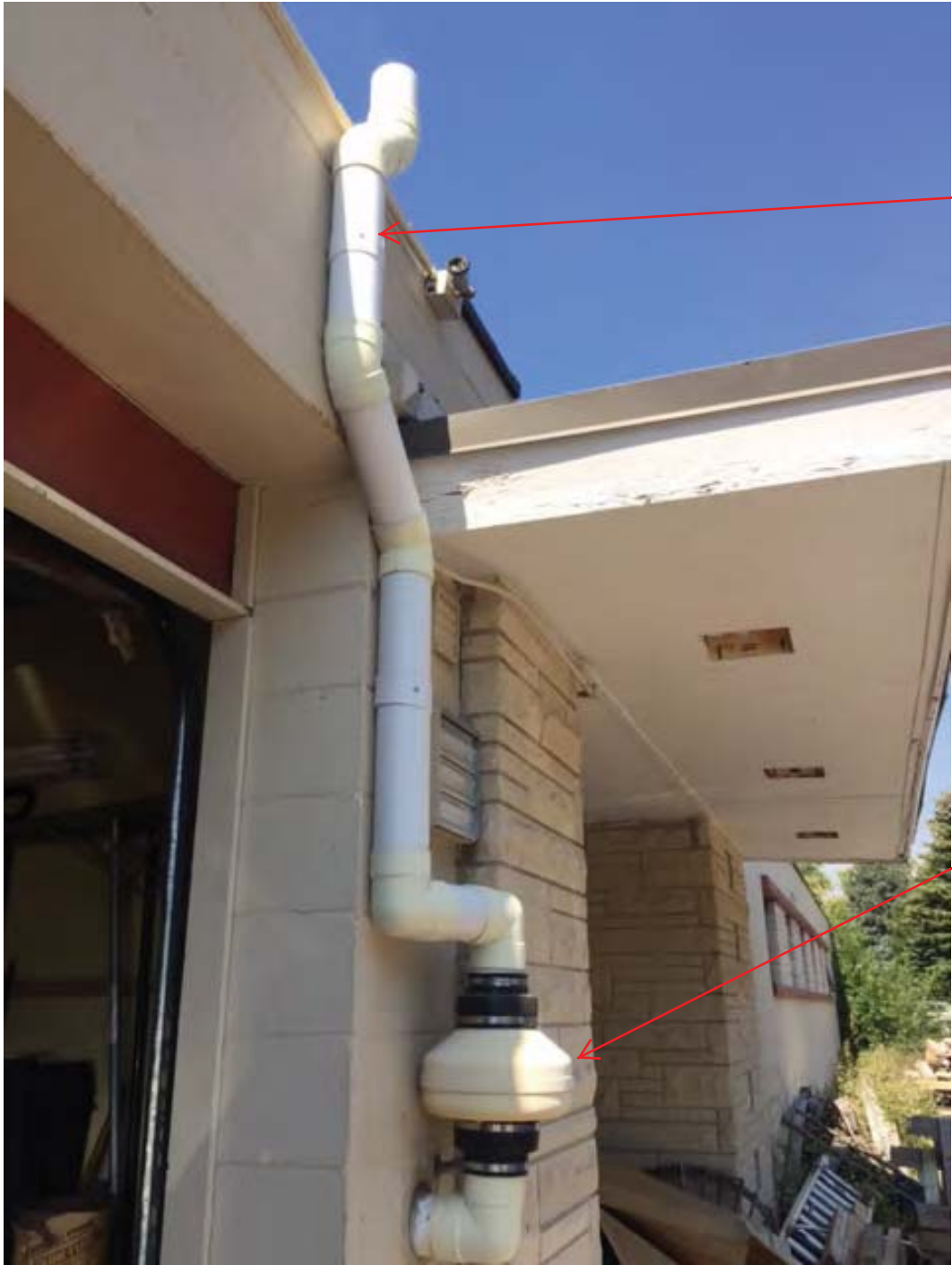
Vapor system located on the east side of the building showing the vent piping going up to the roof line of building.
