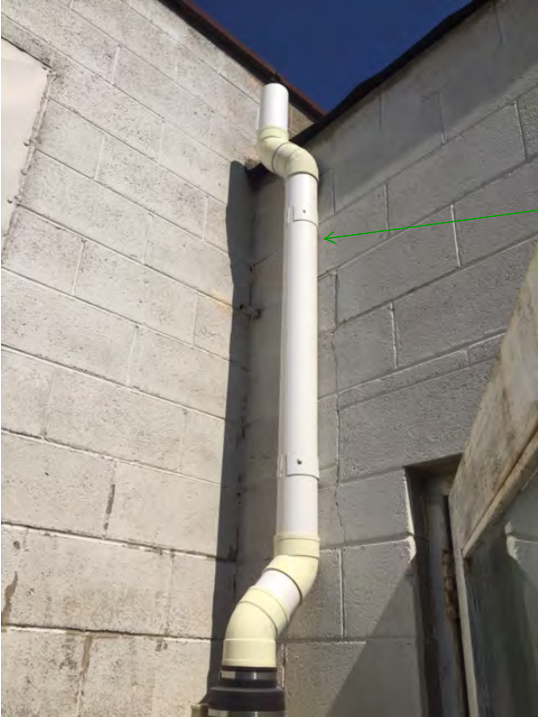
Vapor system located on the west side of the building showing the vent piping going up to the roof line of building.
