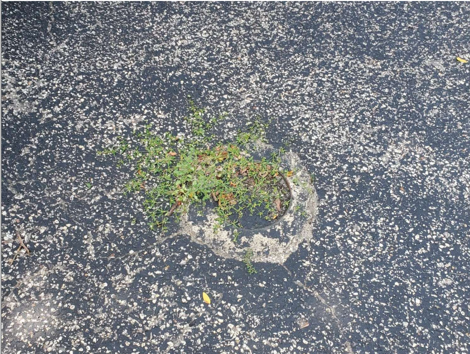
Title: Abandoned monitoring well MW-2
