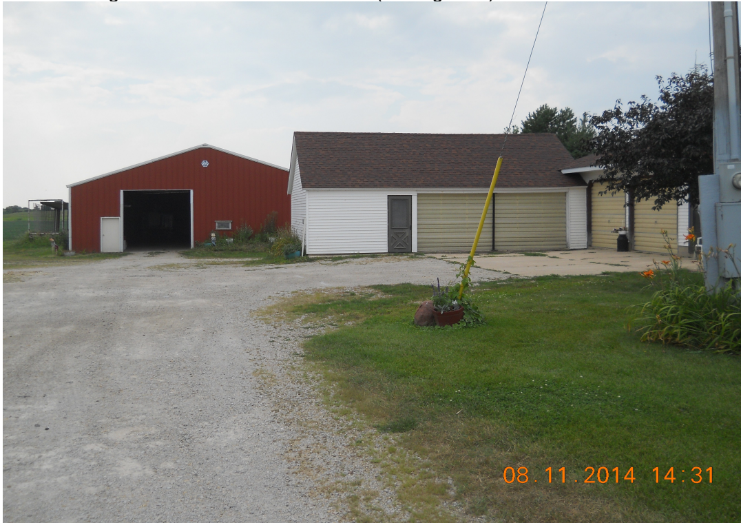
Photo #1: Garage and area of removed UST's (looking west).
