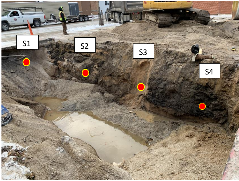
View of tank cavity sidewall sample locations
