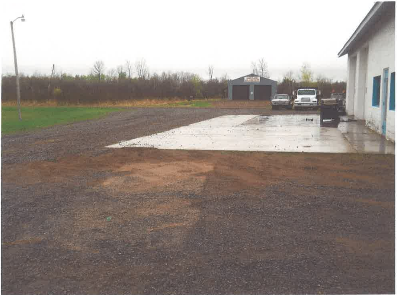
Photo #1: Concrete slab looking west.
