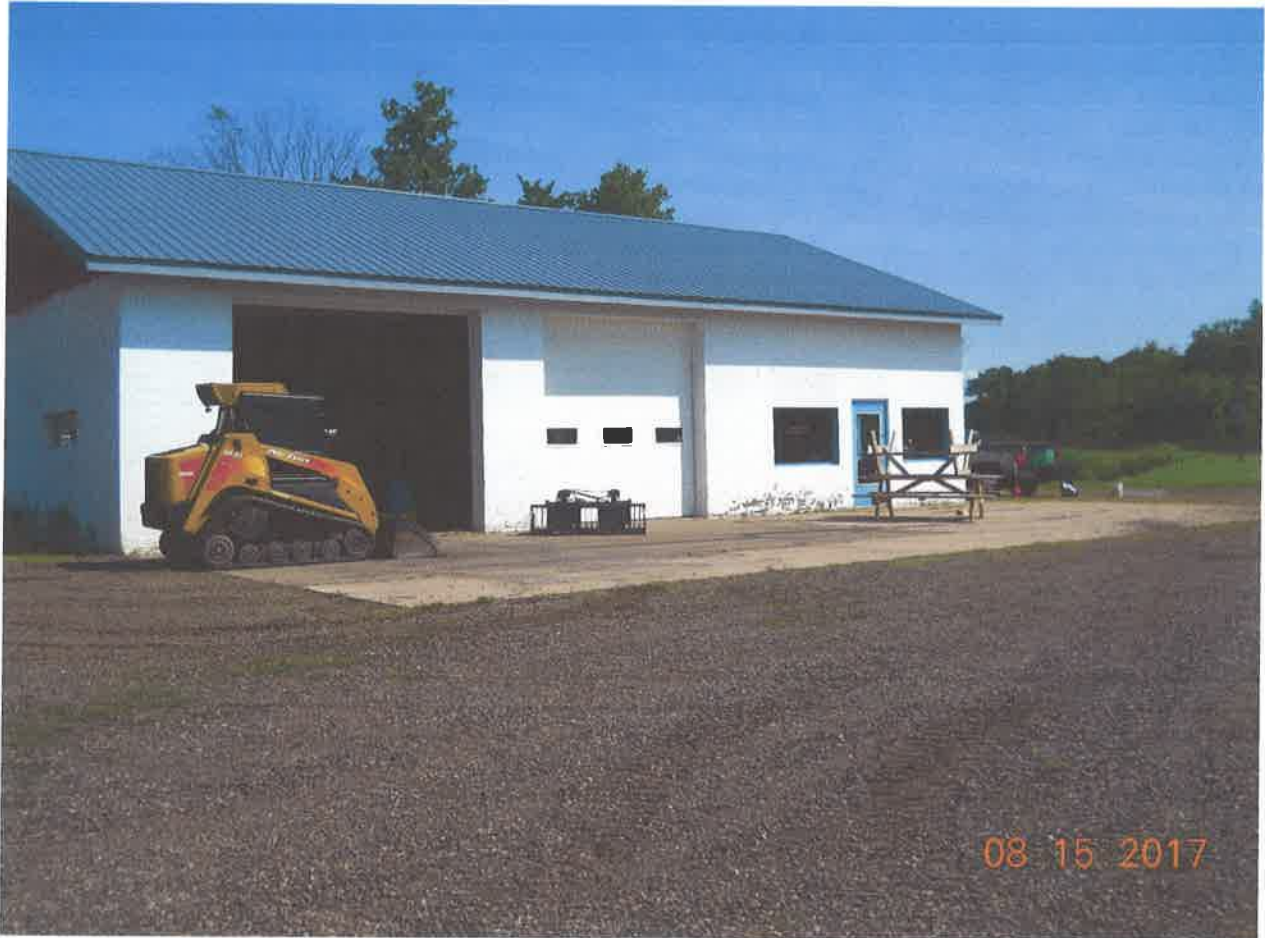
Photo #2: Concrete slab looking northeast.
