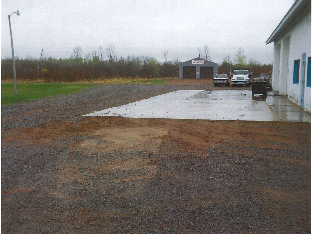
Photo #1: Concrete slab looking west.
