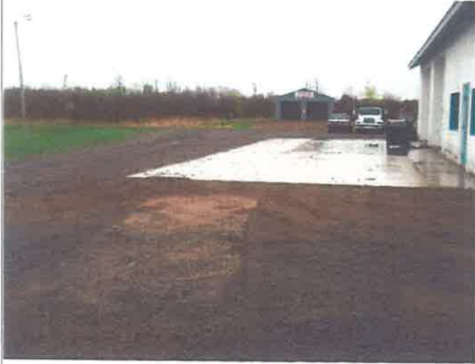
Title: Photo #1: Area of cap to be maintained looking west.
