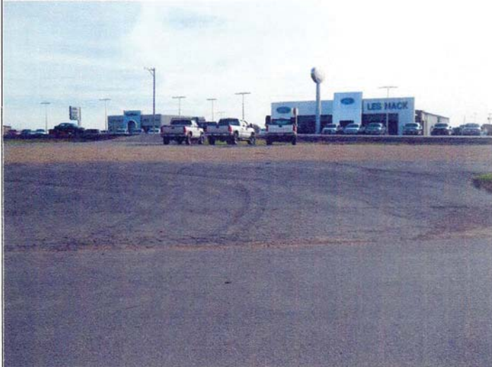
Title: Photo #3: Area of cap to be maintained (looking east)
