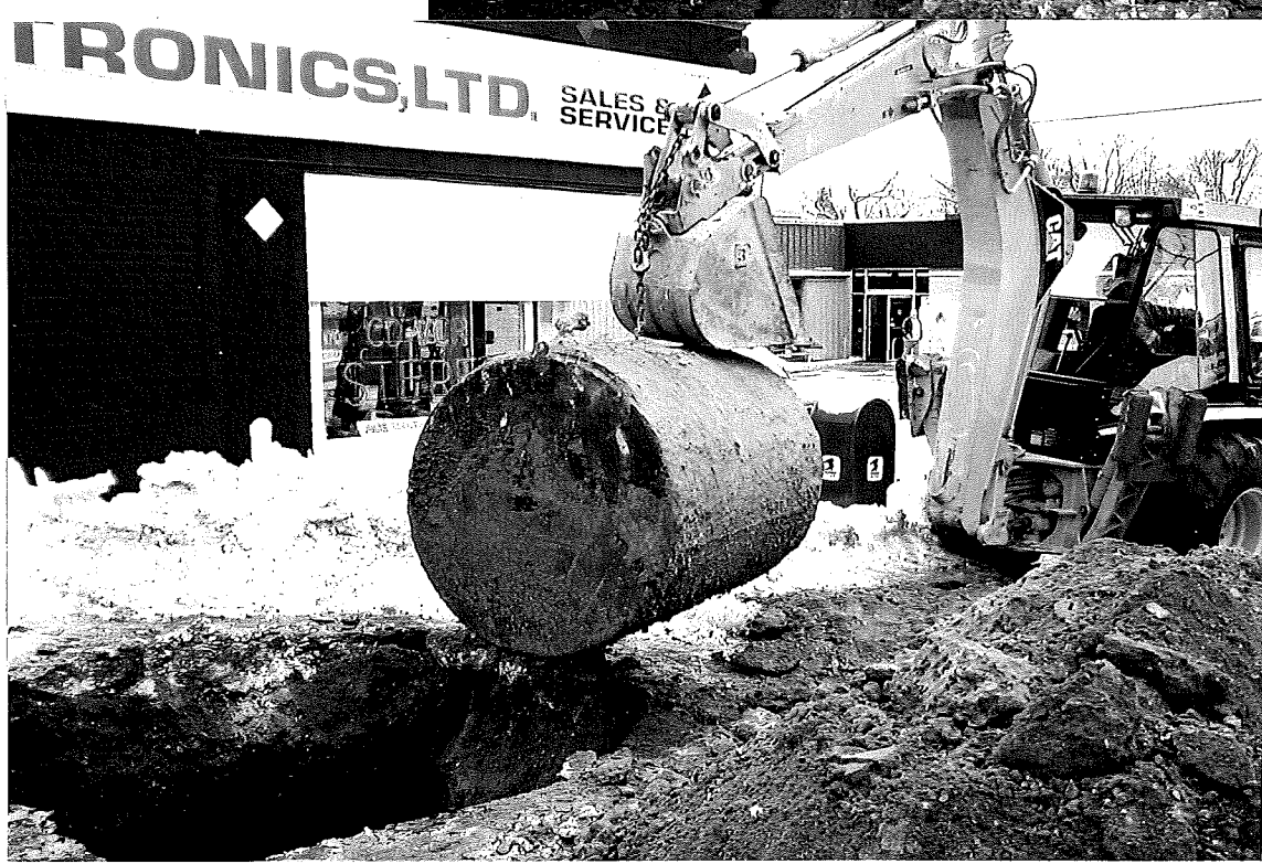
PHOTOGRAPH 2: Removal of the UST from the excavation prior to cleaning.
