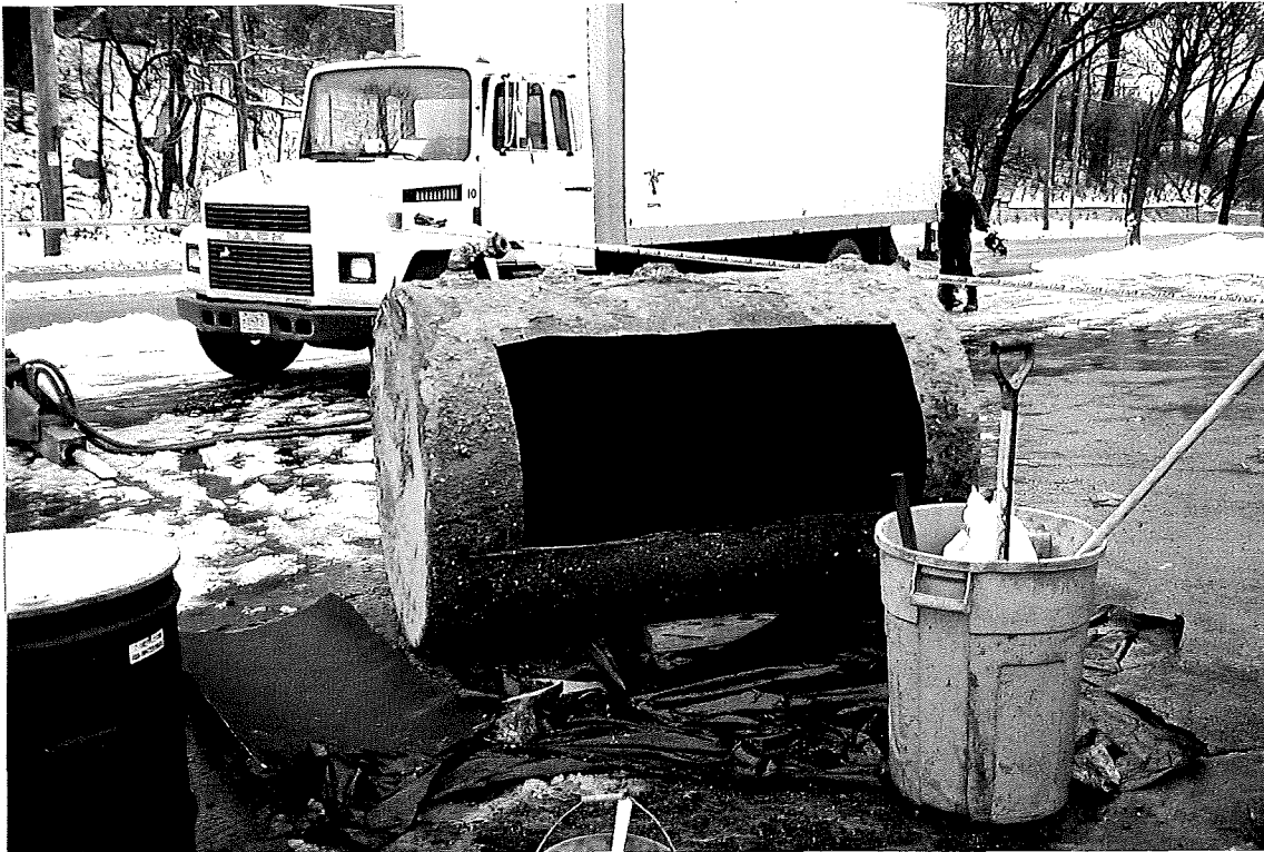
PHOTOGRAPH 3: Opening of the UST to provide access for cleaning.
