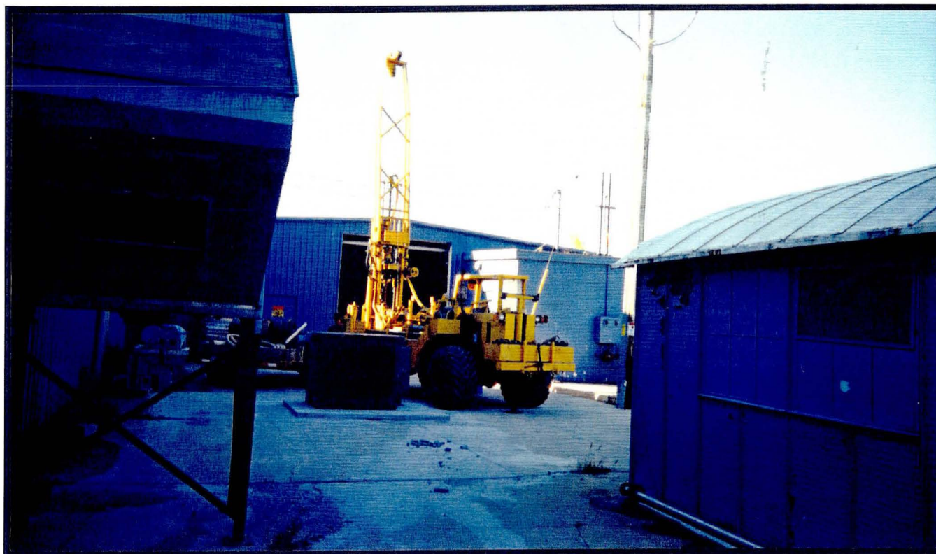
Photograph 1 Drilling of PZ-A (boring B-18), looking South. (September 15, 1999)
