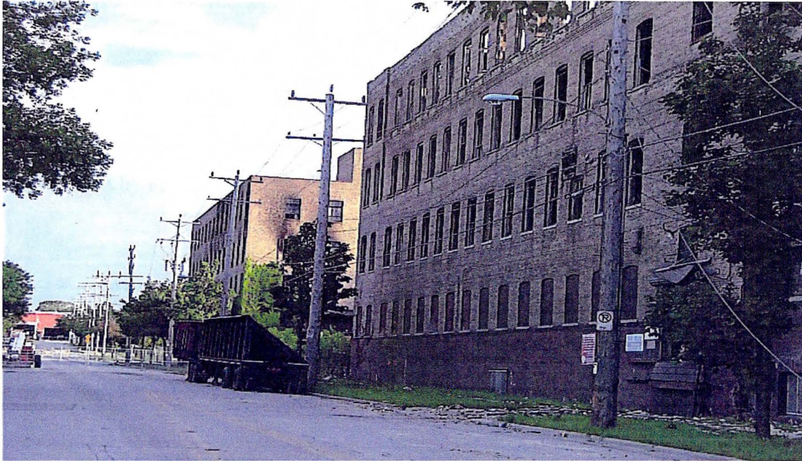
VIEW OF PROPERTY PRIOR TO DEMOLITION
