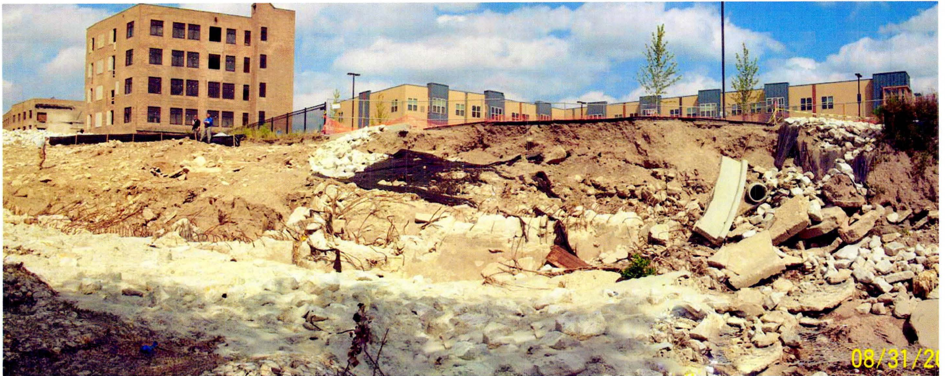
View of bank area flood damage looking north.
