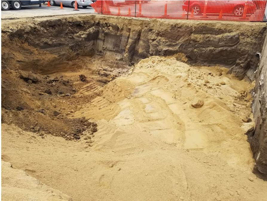
Photo 11: Looking north at backfill from south side of excavation on May 22, 2018.
