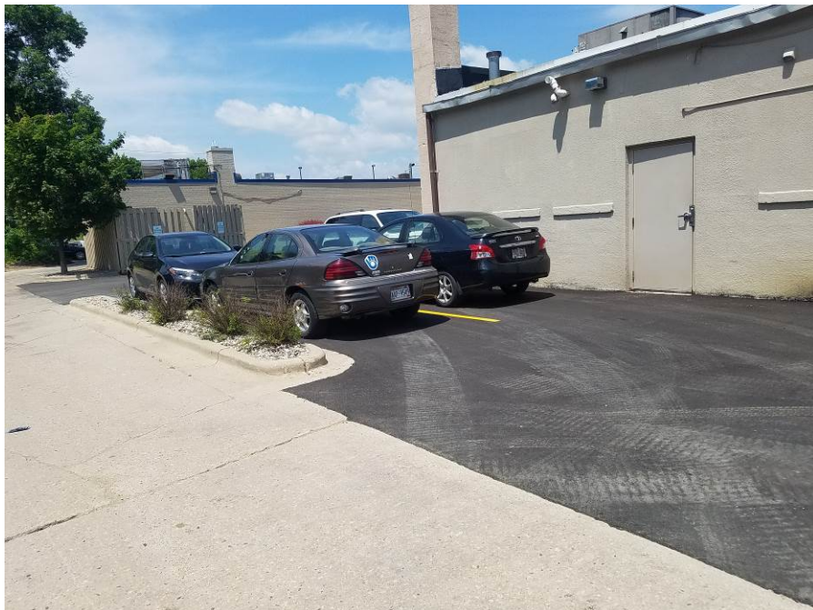
Photo 18: Looking northwest at new pavement at south end of building on June 7, 2018.
