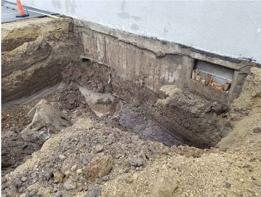
Photo 5: Looking northeast at excavation along west wall of building on May 21, 2018.
