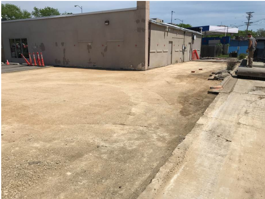
Photo 16: Looking east at southwest corner of building on May 24, 2018.
