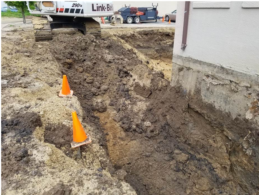
Photo 8: Looking west at excavation from south wall of building on May 22, 2018.
