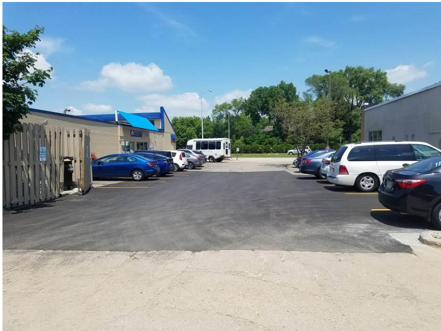
Photo 2: Looking north at pavement and buildings on June 7, 2018.
