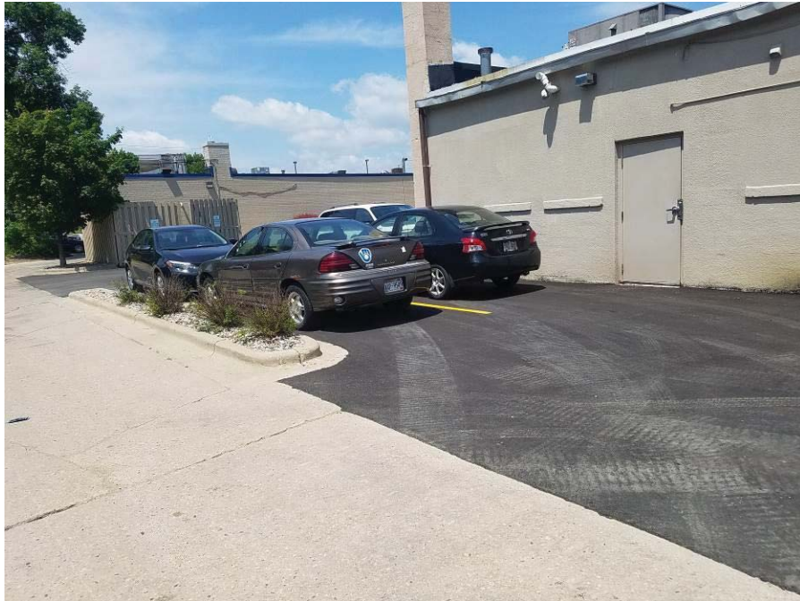
Photo 1: Looking northwest at pavement and buildings on June 7, 2018.
