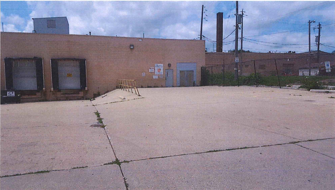
Title: Dock Parcel (Parking Lot), Facing W (7/10/2017) - Findley Adhesives Property, BRRTS #: 03-41-005301
