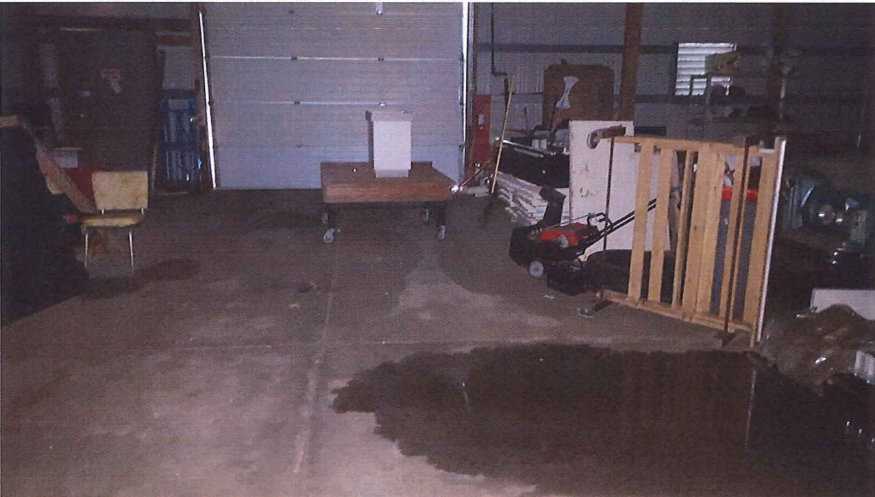
Title: Main Parcel (Parking Garage), Facing W (7/10/2017) - Findley Adhesives Property, BRRTS #: 03-41-005301
