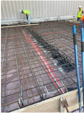
Photograph 5: Overview of Vapor Barrier Installation with Rebar
