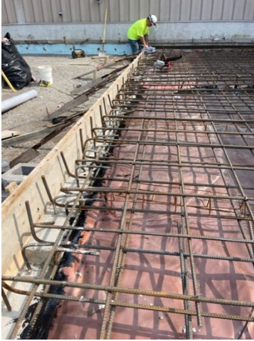
Photograph 3: Overview of Vapor Barrier Installation with Rebar
