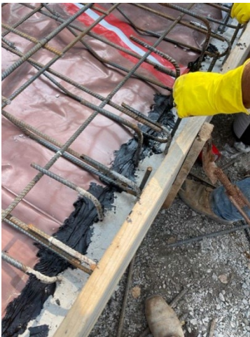
Photograph 4: Close up of Vapor Barrier Installation Along Concrete Foundation
